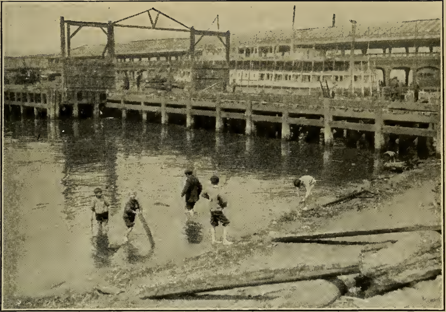
WADING IN SEWAGE LADEN WATER
